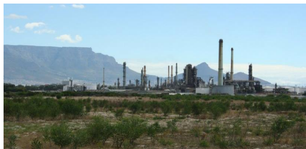
Chevron Oil Refinery, Cape Town, South Africa.
