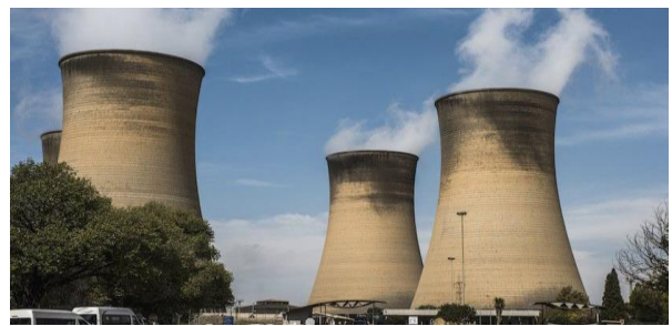
File Photo: Cooling towers operate at the Hendrina power station, operated by Eskom Holdings SOC Ltd. Photographer: Waldo Swiegers/Bloomberg
